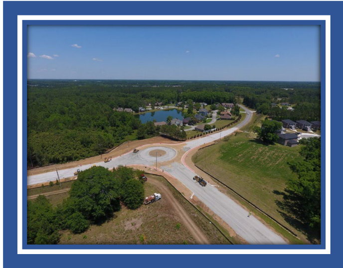
Langston Chapel Roundabout Source: EMC
